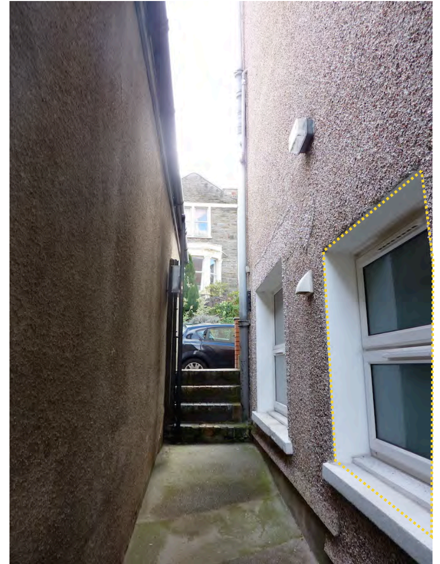
Window location - photo
