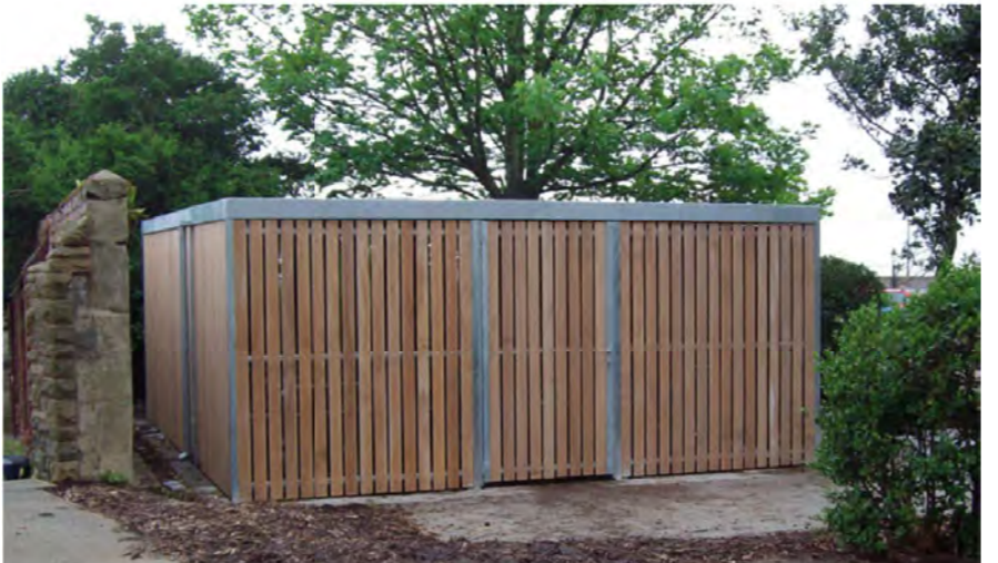
EXAMPLE TIMBER REFUSE/BIKE SHELTER. SHELTERS TO BE COVERED AND SECURE WITH SHEFFIELD STANDS PROVIDED FOR BIKE STORAGE.
