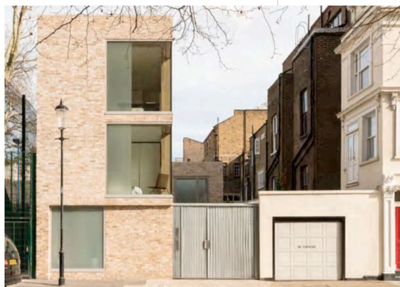
Type of obscured glazing proposed to curtain walling at rear
